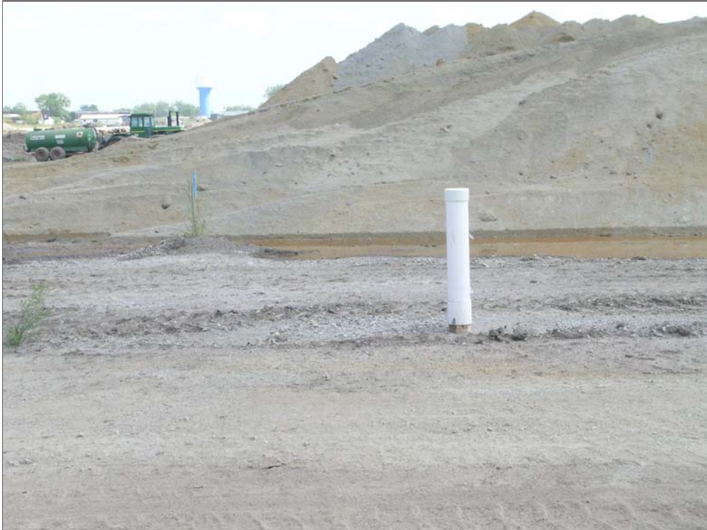
West Commerce project, summer 2006. View looking east with the City of Commerce water tower in background and OCC-5 well in foreground. Chat pile behind the well is part of the 11,000 cy of chat that is planned to be injected into the flooded underground mine voids.
