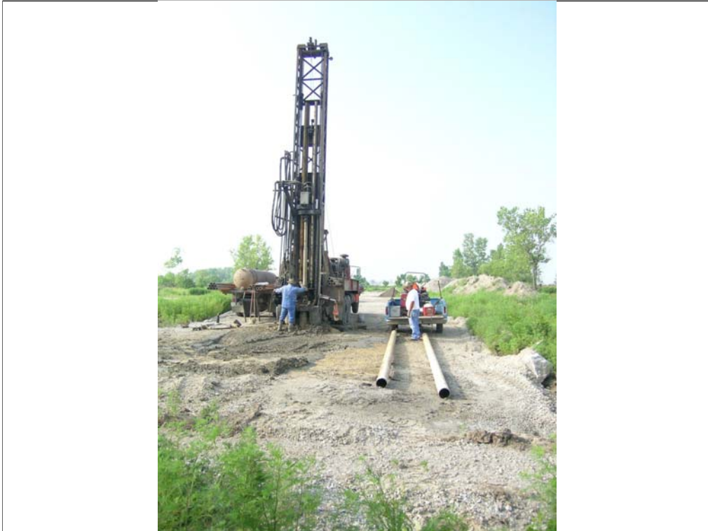
Drilling 6-in exploratory well number OCC-5 on the West Commerce project, summer 2005.
