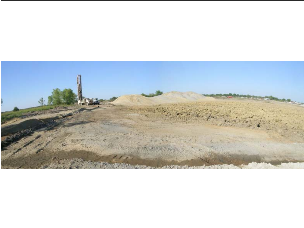
Drilling injection well 5A and view of 11,000 cy yd chat pile to be injected into the mine workings.
