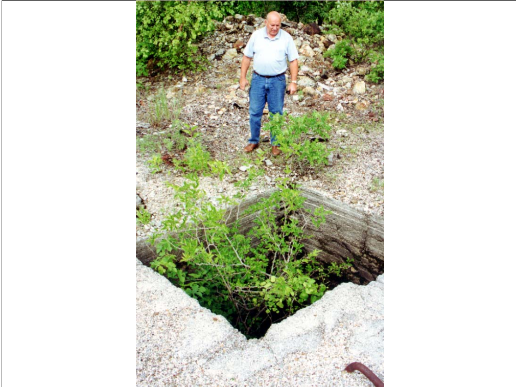
Open shaft in Lead/Zinc mining district. Approximate depth = 250 feet.
